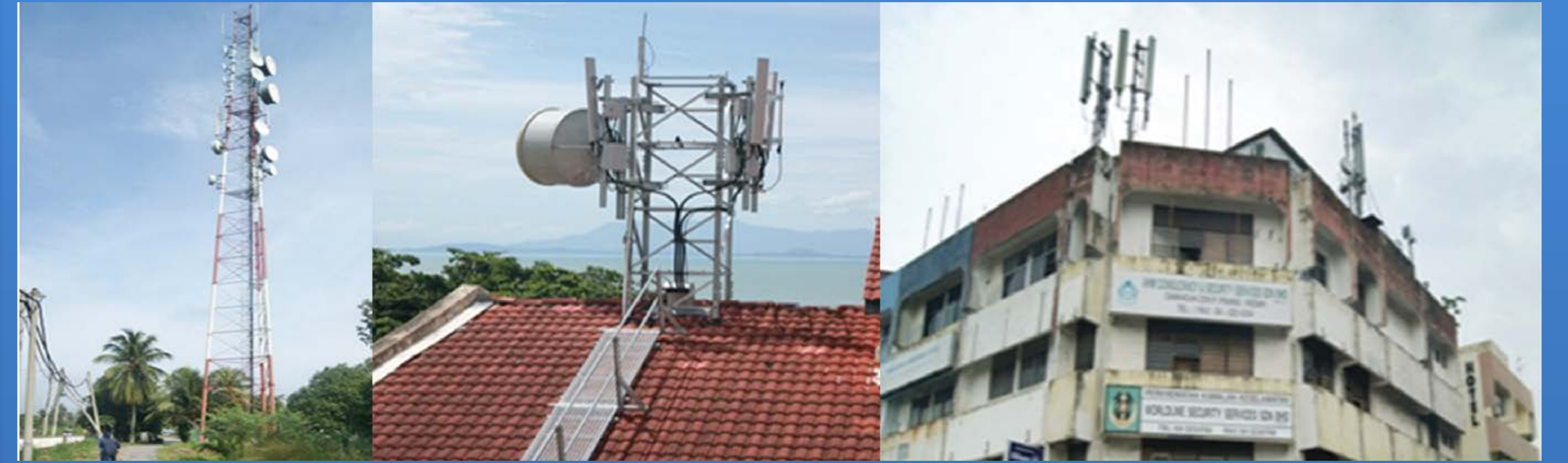
Figure 1: Telecommunication structure located adjacent to residential and commercial area
