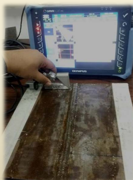
Inspection using Phased Array Ultrasonic
