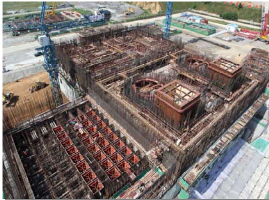
The construction of 7.55 m floor slab
