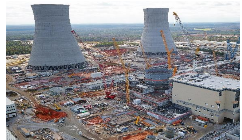
Vogtle Site, Georgia, U.S. Image courtesy of Southern Nuclear
