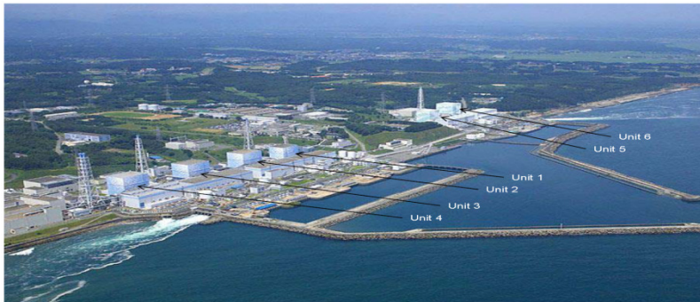
Used by permission from TEPCO
