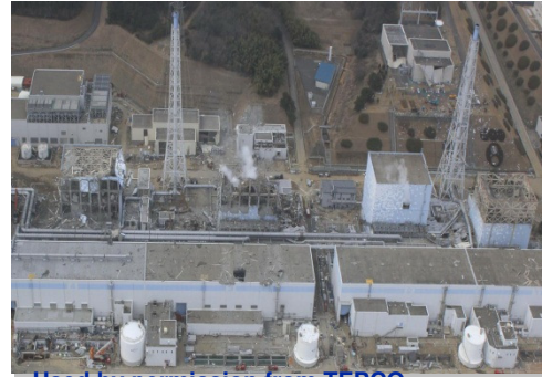
Used by permission from TEPCO
