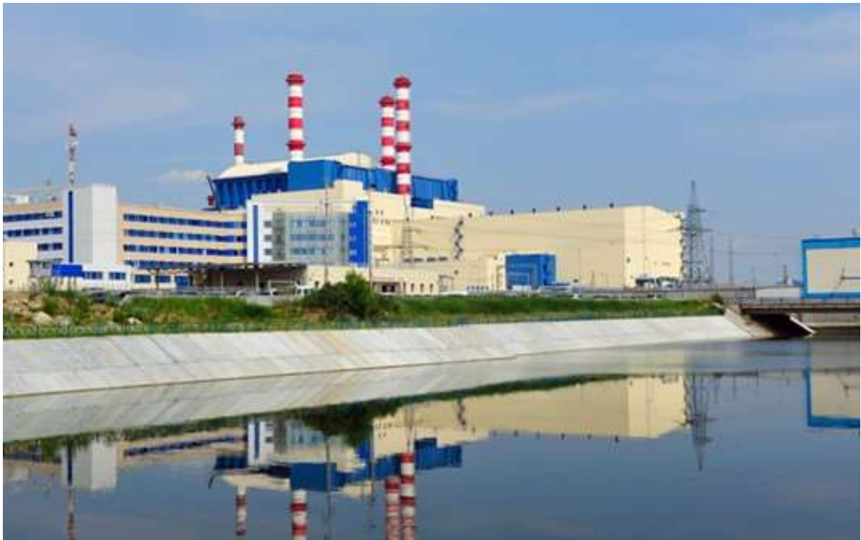
FIG. 1. The BN-800 power unit at the site of Beloyarsk NPP (courtesy of Rosatom).
