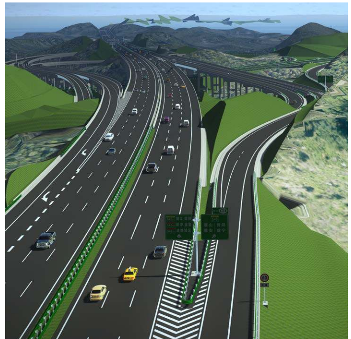
SRB developed a construction management platform and smart beam fabrication system to help save CNY 17.5 million.
