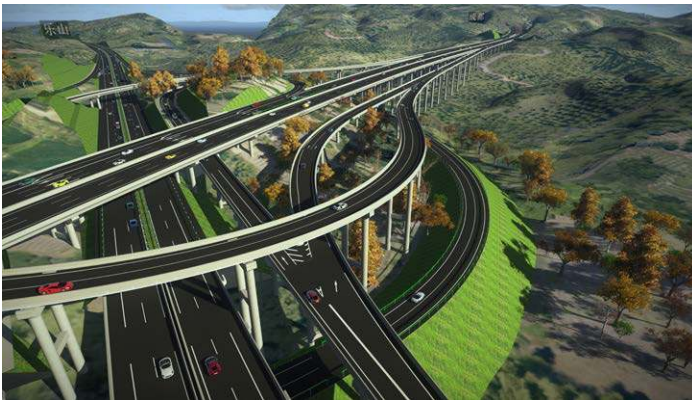
SRB used OpenRoads and LumenRT to model, visualize, and correct line-of-sight issues at the 17 interchanges along the 155-kilometer route.
