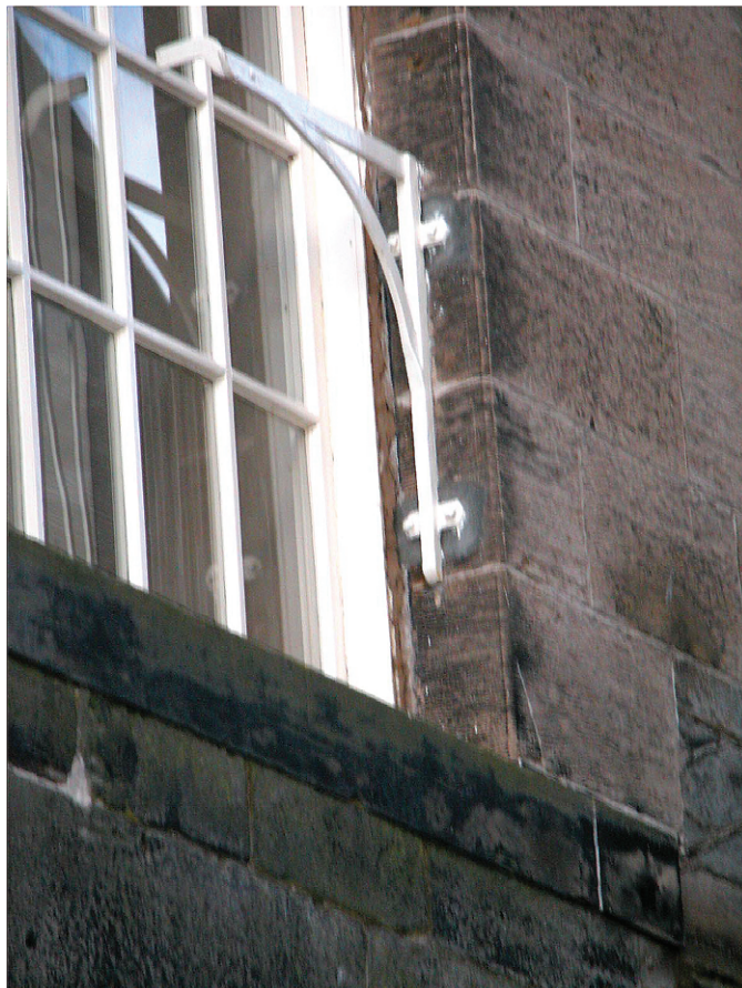
Figure 2. Gregory's telescope bracket placed in one of the southern windows of the rebuilt Upper Parliament Hall as seen from the Quadrangle of St Mary's College. The bracket head is 6.75 metres above ground level
