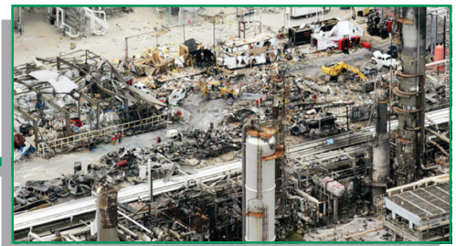
FIG. 10— The aftermath of the BP Refinery explosion.
