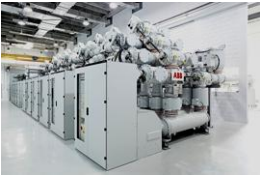
ELK-14, 300 kV duble busbar arrangement
