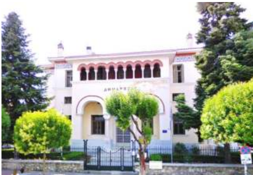
Figure 22 External view of the City Hall building
