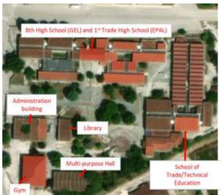
Figure 23 Arrangement of the school complex buildings
