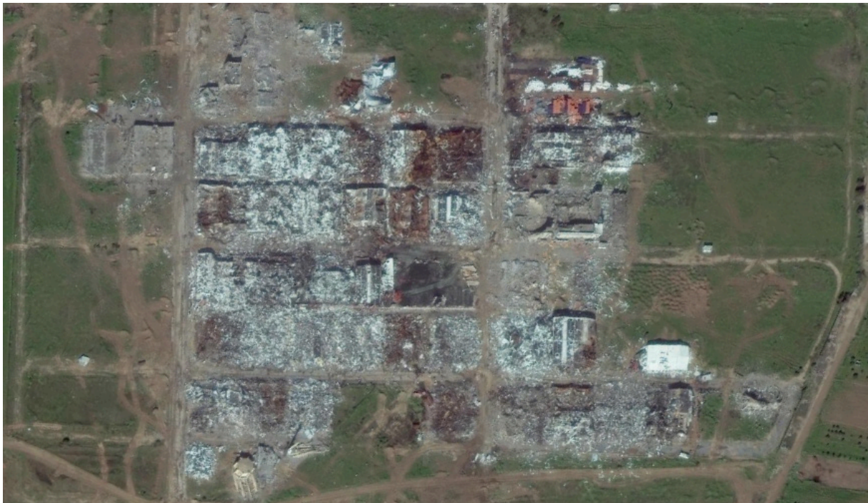
Figure 9. Satellite image showing the complete destruction of the Gaza Industrial Estate (Gaza Governorate). Source: UNOSAT-UNIDO Joint Assessment, February 3, 2024
