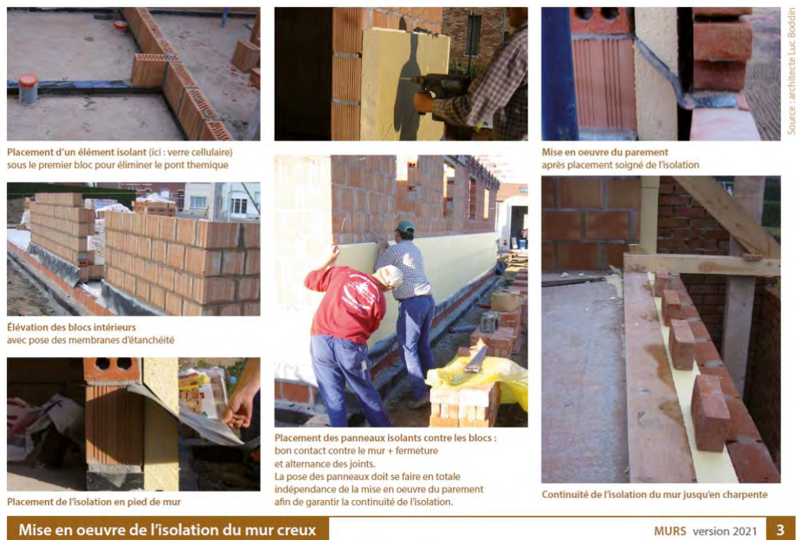
Figure 2: Installation of insulation on site
