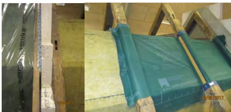
Photos: Demonstration of insulation in Danish training centre
