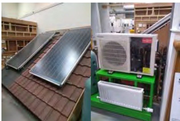
Photos: Solar panel installation and heat pumps at CAVC
