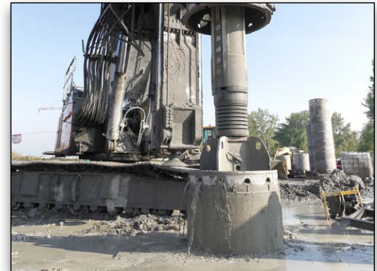
ProjectWise's collaborative environment improved efficiencies and enabled Hatch to complete the detailed design on time and within budget.
