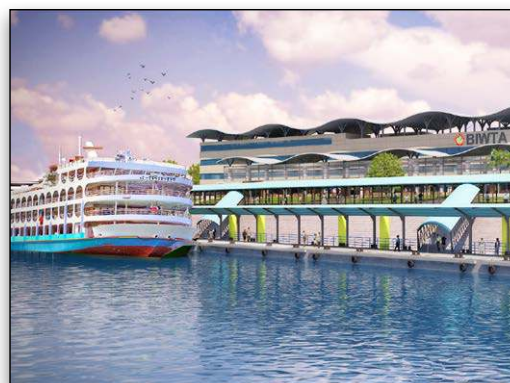
Bentley software was used to overcome structural challenges on the land and marine sides.
