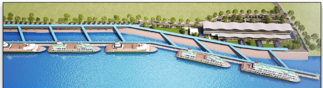
River pontoons and linkspans were designed to withstand water level variations of 6 meters to 7 meters.
