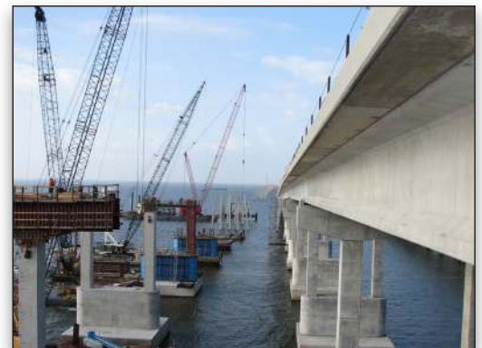
Construction proceeded at an efficient and fast pace.
