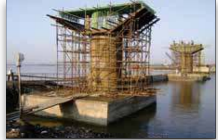
Figure 3: Preparing the Pier Cap Rebar Cage for Concrete Placement
