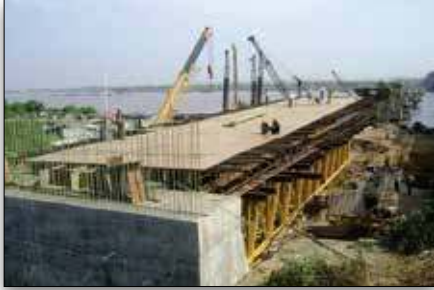
Figure 1: Superstructure Formwork Preparation
