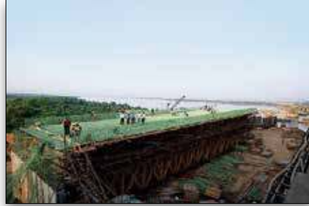
Figure 2: Preparing the Box Girder Rebar Cage for Concrete Placement
