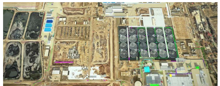
PC3 leveraged SYNCHRO and iTwin to develop a digital twin to manage 22 engineering projects on an active wastewater treatment plant.
