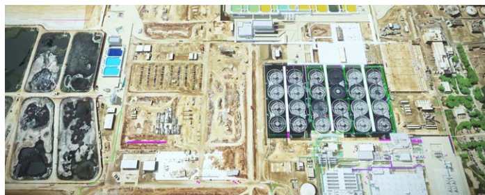
Regional San initiated the decade-long EchoWater facility upgrade to provide safe and reliable treated water for recycled water use.
