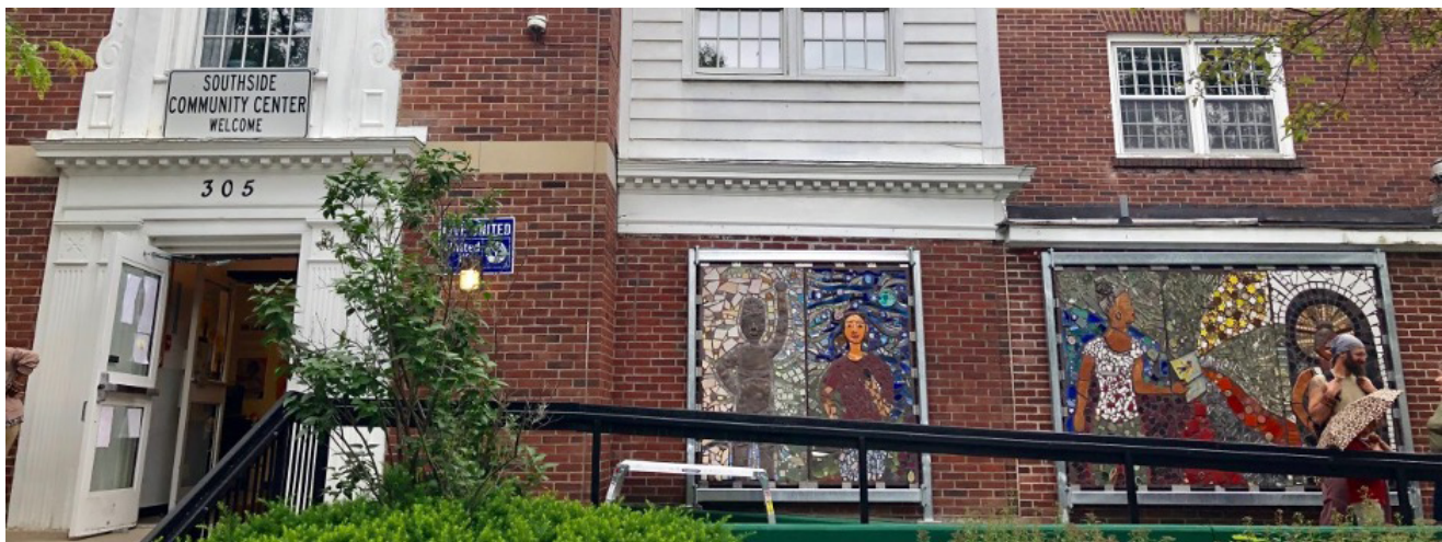
South Side Community Center, one of the first buildings slated for retrofits in Ithaca.
