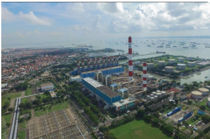
Gresik Power Station
