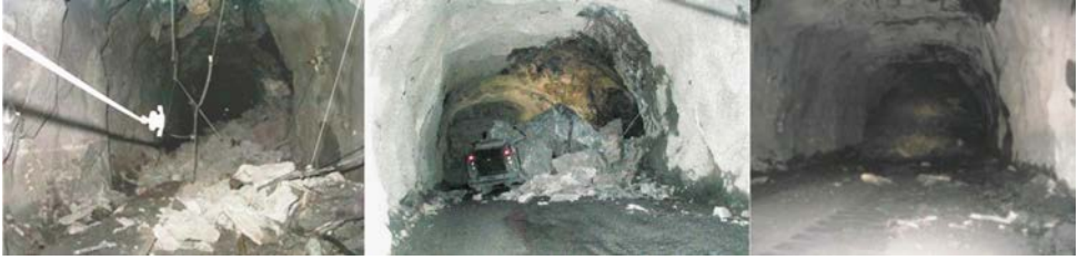
Figure 5.1: Examples of rockfalls after seismic events in the underground mines [152]
