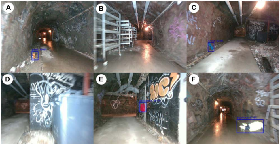
Figure 5.11: COMPRA mission in an obstacle filled tunnel section and critical moments during the mission. (A), (C), (E), (F) shows artefact detection hits while (B) and (D) show collision avoidance situations during the mission.
