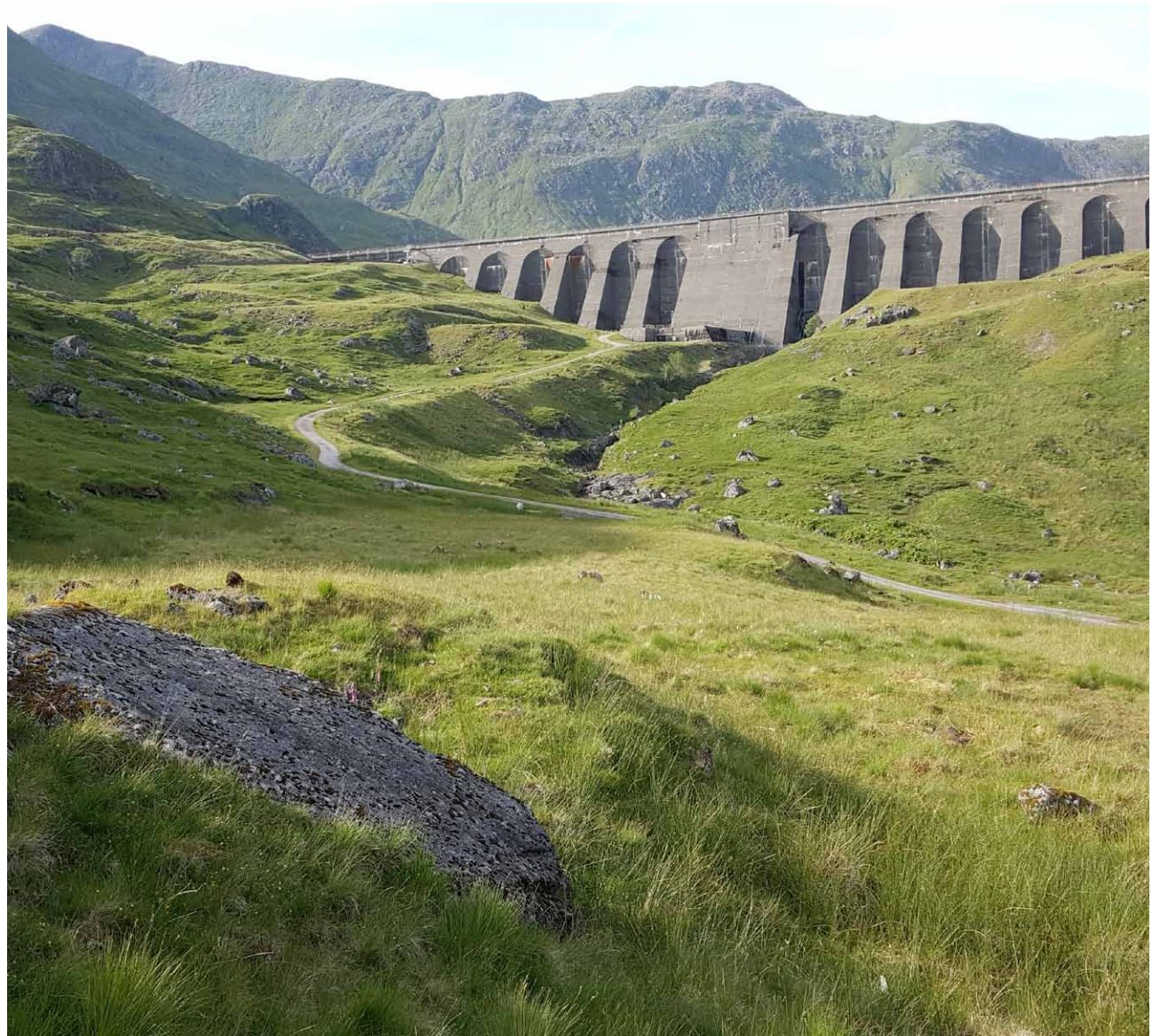
Looking northeast towards Cruachan Reservoir and its buttress dam with the west side access road in the foreground
