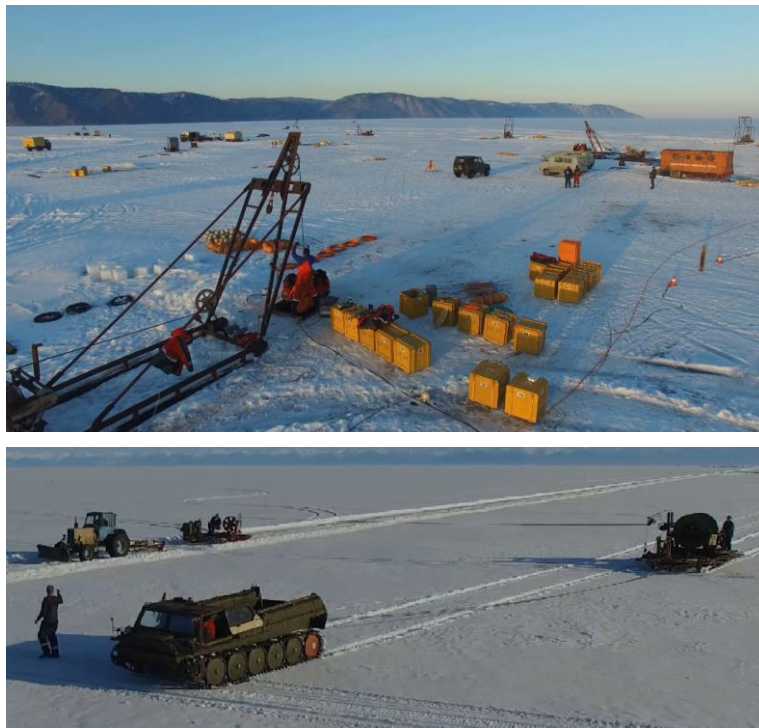
Figure 2. Ice camp (top) and cable laying equipment (bottom).
