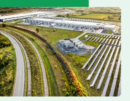
During day-to-day data centre operations, the main generators of noise are external cooling plants, on-site substations, and miscellaneous HVAC equipment. To mitigate the impact of this noise, Google adjusts designs for cooling towers closest to residential areas and only conducts unavoidable maintenance of equipment like generators during the day.
