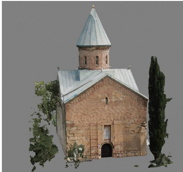
Figure 11. Textured and meshed 3D model from PhotoScan (Alignment "medium", Dense cloud "high", Mesh "arbitrary, high", Texture "adaptive orthophoto, mosaic")
