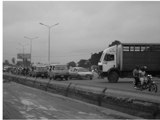
Fig 5: The truck marked B cannot make a u-turn in one go. Notice that there is congestion resulting from blocking of the road
