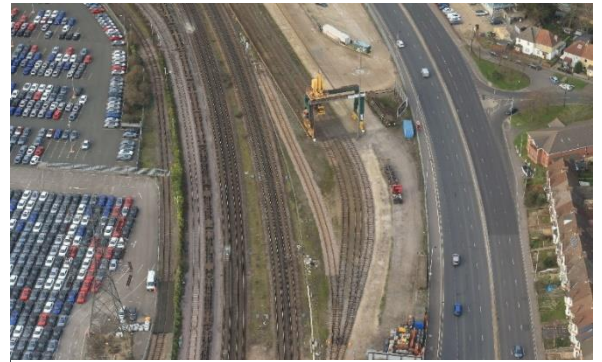
Figure 17 - Millbrook Freightliner Terminal (Source: Network Rail)
