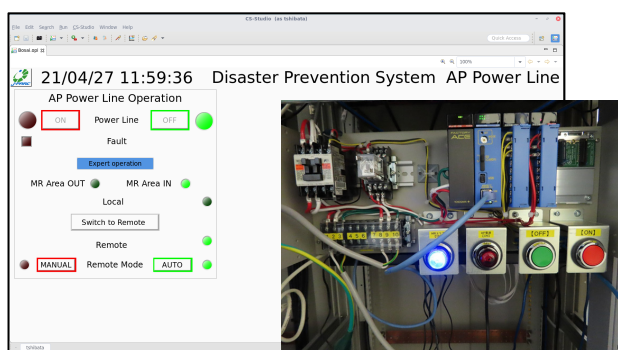
Figure 8: AP power line ON / OFF Controller.
