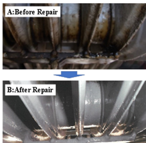
Figure 3: Repair of the radiator. A: before repair, B: after repair.
