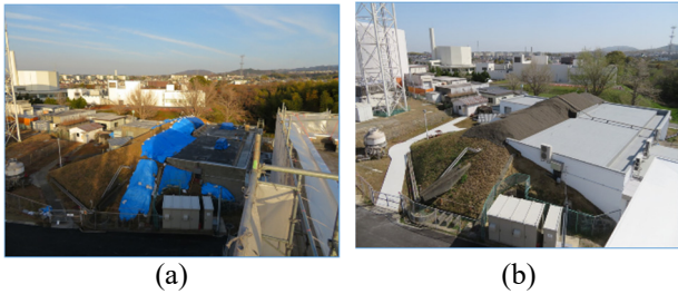
Figure 7: (a) Under repair. (b) Complete repair.
