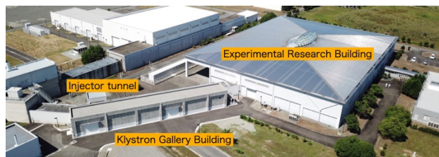
Figure 1: NewSUBARU synchrotron light facility.
