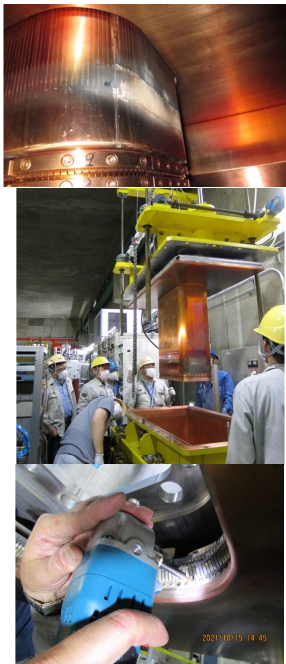
Figure 4: Photo of RFQ being repaired. (top) Damaged area of a shorting plate. (middle) A shorting plate is being lifted by a crane for the repair. (bottom) New contact fingers are attached to the shorting plate.
