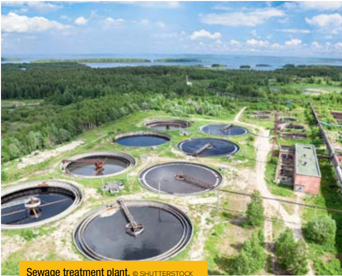
Sewage treatment plant. © SHUTTERSTOCK
