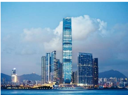
Kowloon Station in Hong Kong
