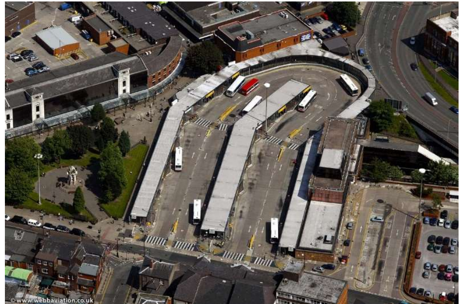
Interchange integrating Metrolink LRT and Bus services
