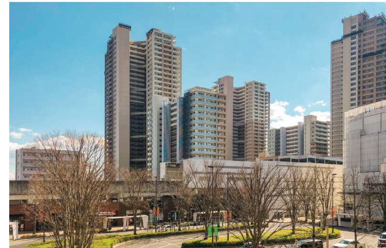
Tsukuba Express, Kashiwa-no-ha Campus Station Area
