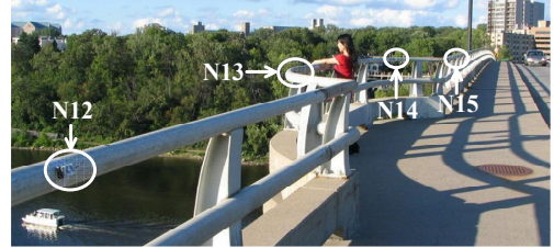
(b) On-site View
